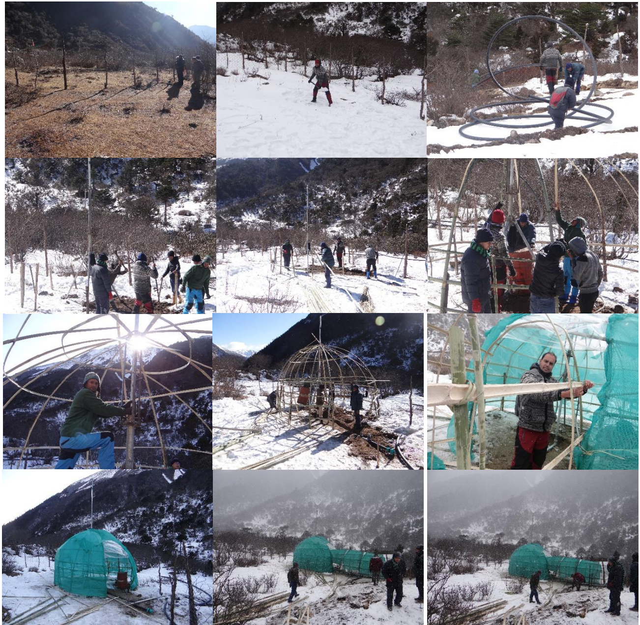
Fig. Stepwise detail photographs in making of Ice Stupa at the site
